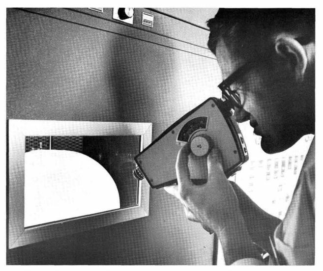
CHECKING THE TEMPERATURE in the epitaxial reactor with an optical pyrometer is Vic Wells (2141). The system is used for chemical vapor deposition of materials used in the fabrication of semiconductor devices. Availability of the reactor provides the Microelectronics Lab with the processing capabilities required for such advanced technologies as silicon gate and MNOS integrated circuits.
